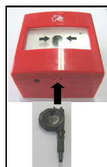
Picture 10 - front device block removal from its wall mounting back box
